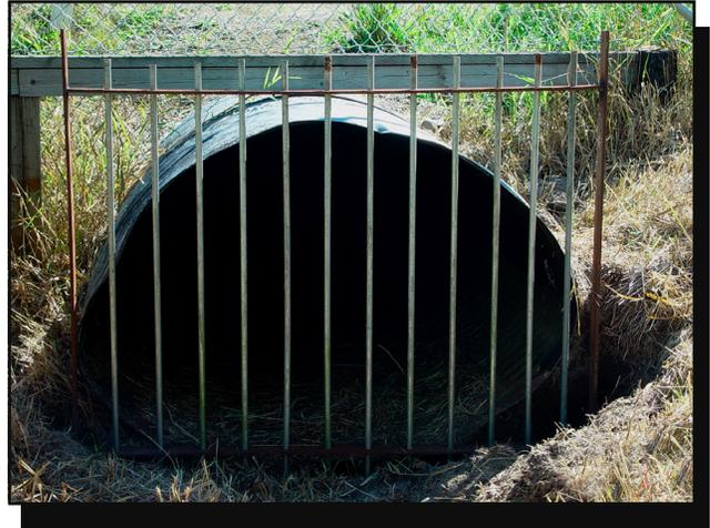
Figure 5—This beaver guard is constructed by inserting steel rods through a frame mounted on the front of a culvert.
