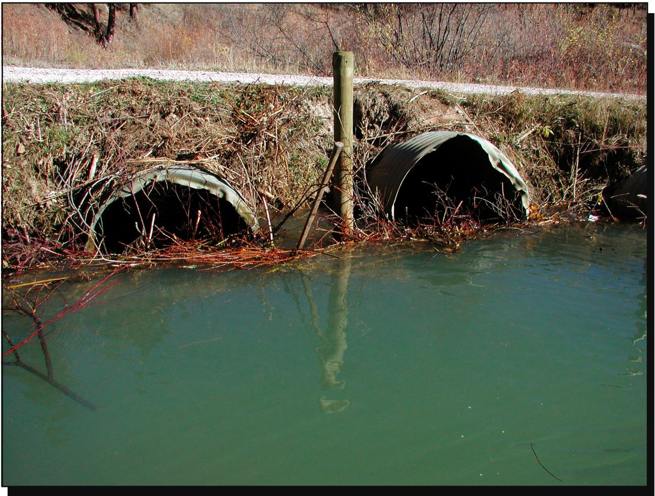
Figure 4—Most culverts create ideal locations for beavers to construct their dams.
